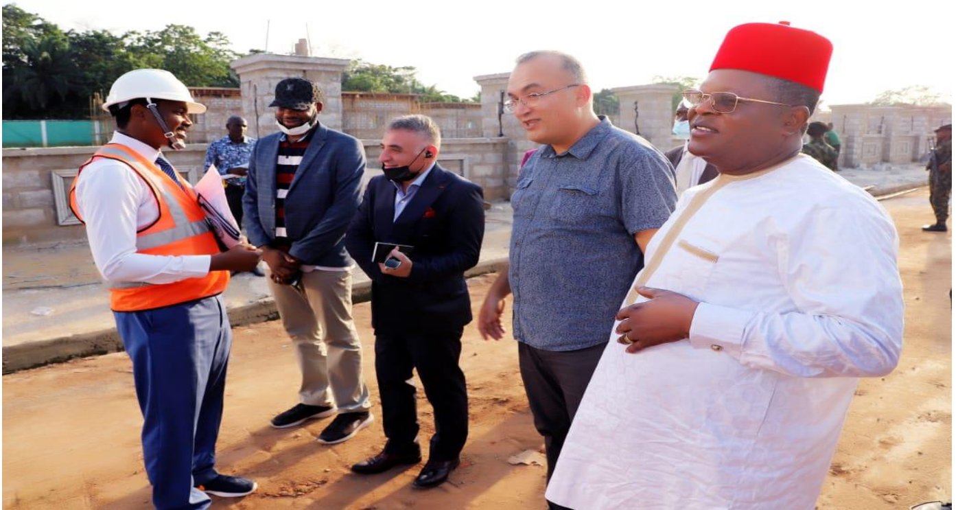
Figure 34. The Vice Chancellor welcoming His Excellency Engr. David Umahi along with visitors from Nile University Abuja at the University premises during the construction of the Facility
