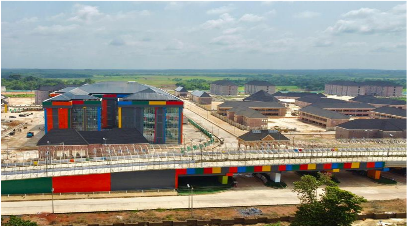
Figure 23. Aerial view of the Main University Block and Students Hostel Blocks
